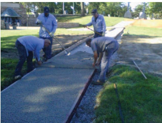
FIGURE 8 SAP mixture: striking off with straight edge.
