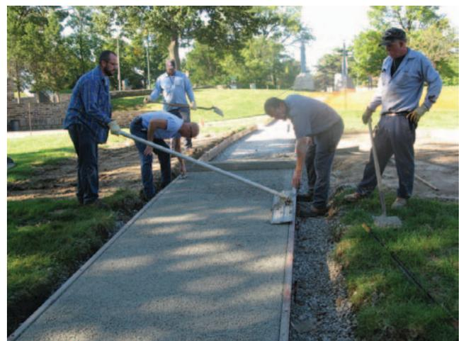
FIGURE 9 SAP mixture: finishing with bull float.
