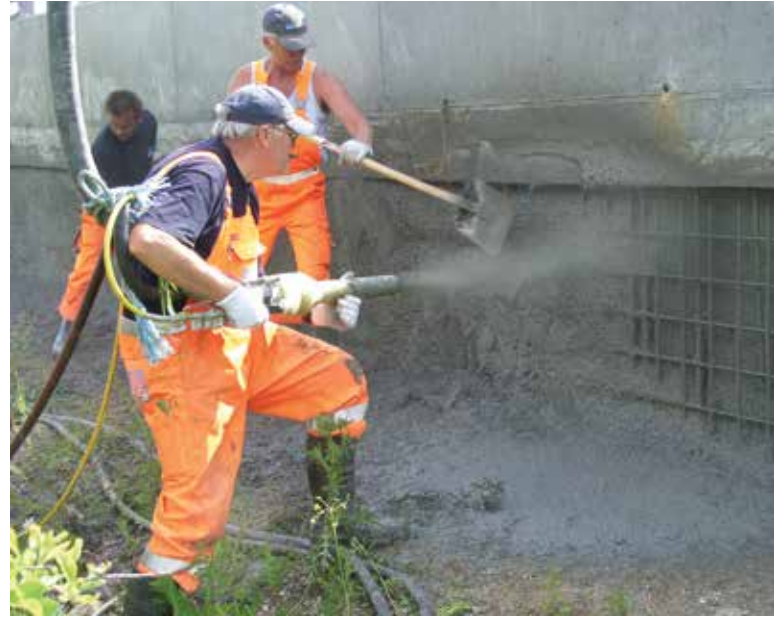
Fig. 5: A nozzleman places shotcrete incorporating SAP as a rheology-modifying admixture
